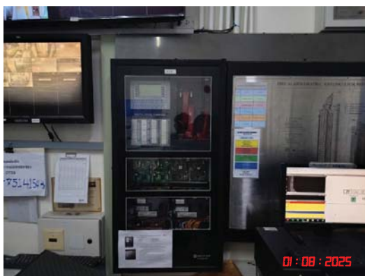
Fire alarm control panel
